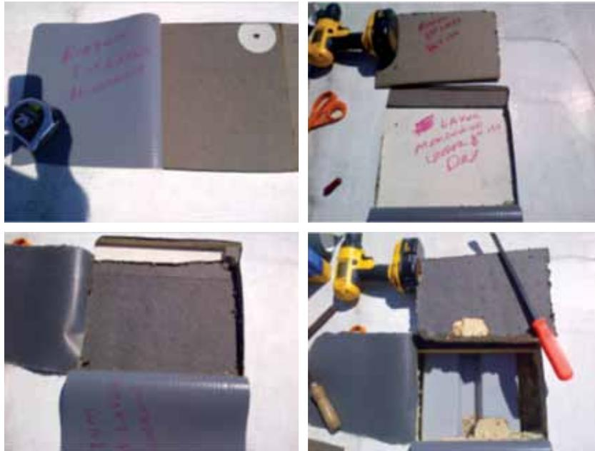
**(TOP LEFT) PHOTO 1:** Cheektowaga, N.Y., top membrane recover board interface. **(TOP RIGHT) PHOTO 2:** Cover board original membrane interface. **(BOTTOM LEFT) PHOTO 3:** Original membrane insulation interface. **(BOTTOM RIGHT) PHOTO 4:** Steel deck.
