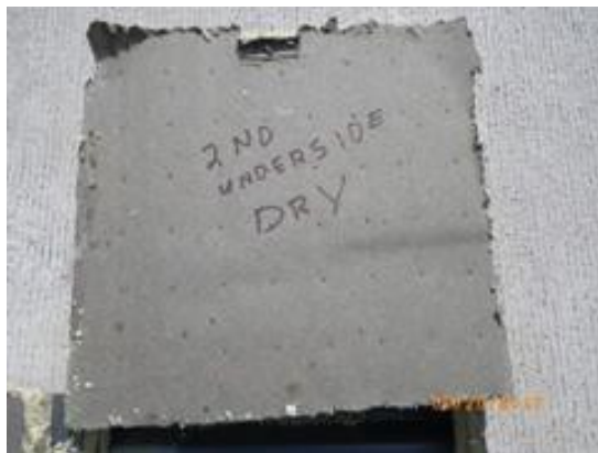
Photo 9: Bottom insulation underside
