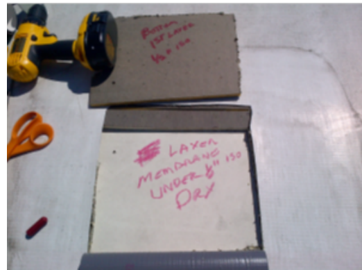
Photo 2: Cover board original membrane interface
