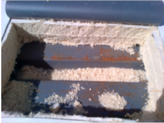
Photo 13: Poughkeepsie, NY Localized rust on deck
