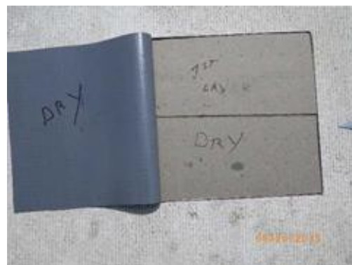
Photo 6: Chaska, MN Membrane top layer insulation interface
