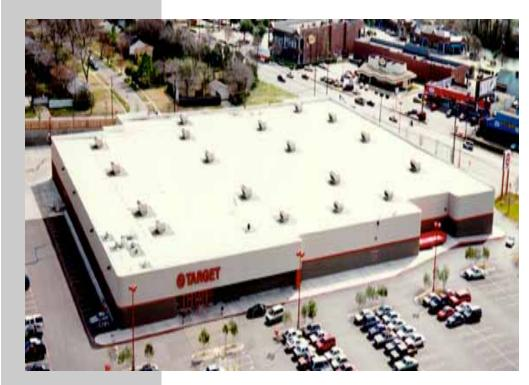
In 2000, the U.S. Department of Energy and the Environmental Protection agency conducted a study where a large retail store replaced a 100,000 sq. ft. black EPDM roof with a white PVC roof. The study confirms that the roof membrane reduced average summertime air conditioning peak demand (1-4pm) by 14 percent and the total daily air conditioning energy usage by 11 percent.
