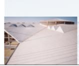
A failing low-pitch shingle roof system on three elementary schools joined by a central rotunda in Plano, Texas, was replaced with the leak-tight security of hot-air-welded vinyl. The light gray reflective membrane formed tight seals around the rotunda's complex curvatures, and rib-like extruded profiles were adhered to replicate the appearance of standing seam metal.
