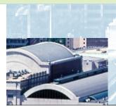
Watertight, UL-listed vinyl membrane was selected to protect the structural and historical integrity of Washington, D.C.'s Union Station. Rehabilitation of the arching barrel roof without ruining the priceless suspended plaster ceiling underneath or old cement falling on the shoppers and travelers below were key requirements.
