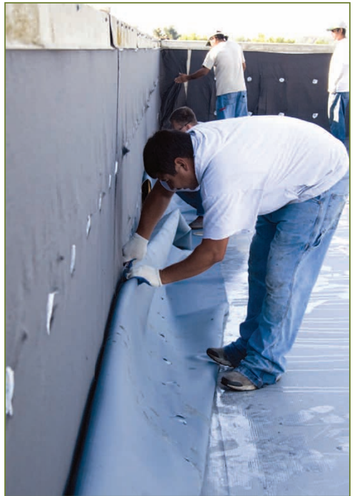
Contractors separate the vinyl membrane from the wall fasteners and plates, which will also be recycled. Image courtesy Vinyl Roofing Division, CFFA.
