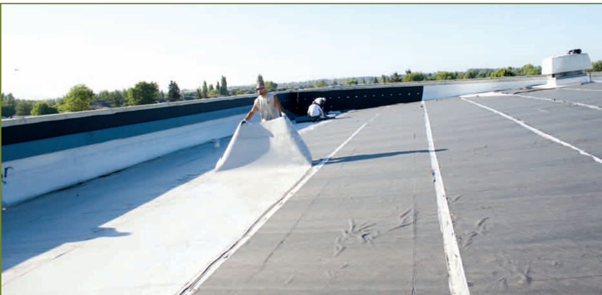
Contractors easily lift a flexible sheet of retired membrane from the roof to be rolled in preparation for transport off site. Image courtesy Vinyl Roofing Division, CFFA.
