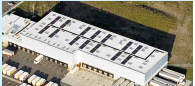
The Frito-Lay Distribution Center in Henrietta, N.Y., incorporates a vinyl roofing membrane and a building integrated photovoltaic (BIPV) solar electric roofing system.
