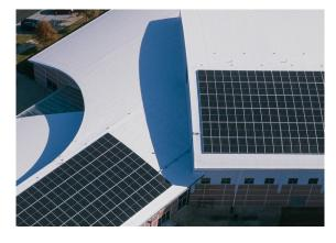
drip edge, fascia, reglet, edge extender and gutters from EXCEPTIONAL Metals were installed around the perimeter to terminate the membrane and complete the primary re-roof portion of the project.
