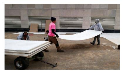
Imperial Roofing out of Iowa was the contractor that executed the project. Imperial removed the original PVC membrane, packaged and bundled it for the recycler to pick up. Approximately 39,000 lbs. (19.5 tons) were avoided from landfill and reused back into roofing products. Imperial, then installed the recycled hard board containing PVC and fluff and then installed the new Sarnafil PVC roof membrane that contains an average of 10% recycled content.
